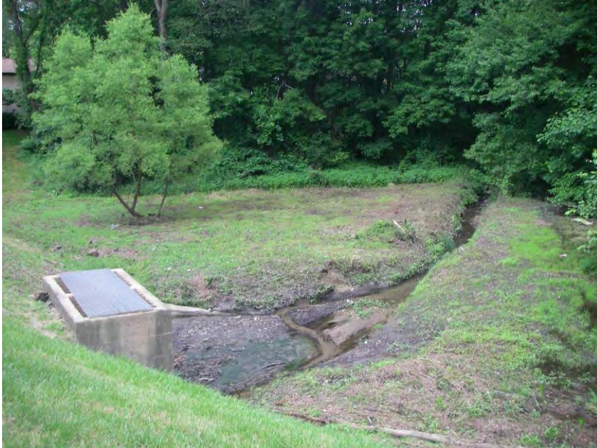
Site Photo: Existing Facility Overview
